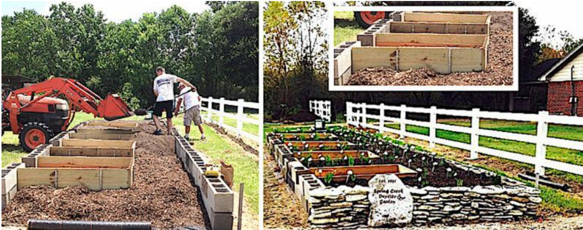
Left, Mary and Eddie Gage's "Smart Garden" under construction and planted. Right, note the insert -- access "openings" for easy reach into the far right side of the beds.
